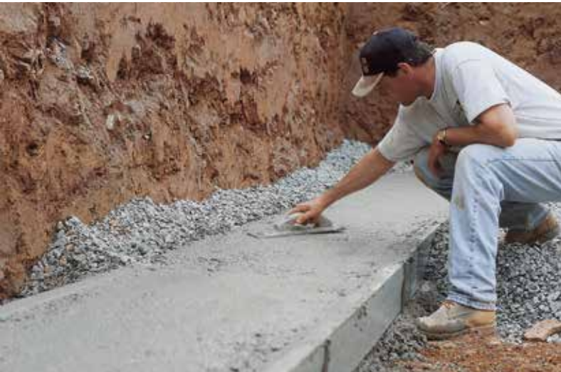
During the concrete pour, grade stakes hold the Form-A-Drain Plus system at the proper elevation. Thereafter, Form-A-Drain Plus remains permanently in place.
