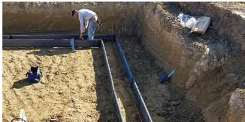
Lineal sections, couplings and corners ensure precise form set-up.
