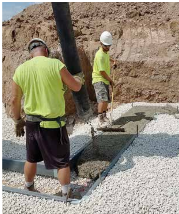
Form-A-Drain installation
