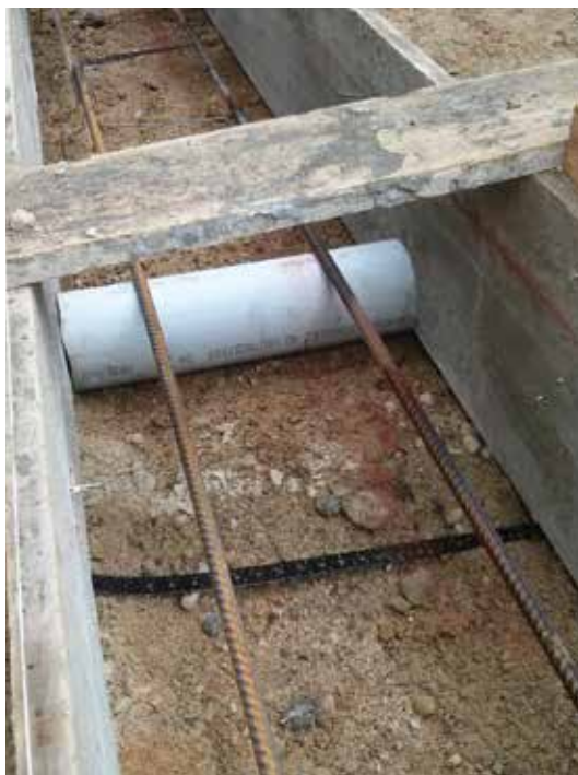
Traditional wood form installation
